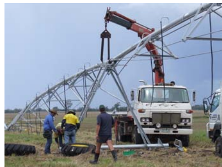
Gavin Bartel, Moree erecting a new centre pivot in 2011. Image J Montgomery
